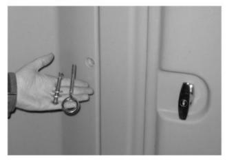
Replace the existing 3/8" mid wall bolts with 3/8" X 5" eye bolts. Reuse the existing nut and washers.
