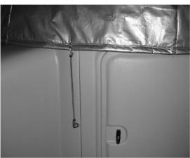
Use a 15 -18" bungee cable to secure the cover to the POD.
